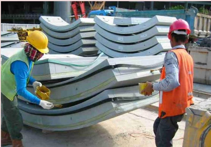
After mounting the gasket, the tunnel segment can be stored outdoor. EPDM is not susceptible to normal weather influences such as sun and rain. But in case of co-extruded profiles with hydrophilic layer, the gasket should be covered with a plastic to avoid swelling before installation of the segments. Most contractors pile segments for a whole ring and protect this set with a plastic cover from possible rain.
